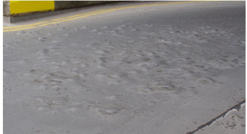
Blisters are caused by trapped moisture and air heating up to create a vapour pressure. This moisture may be in the substrate beneath the asphalt or between the asphalt layers (interstitial) in multi-layer systems found in car parks. The blistering can occur soon after installation, or in some cases, take many years to form. The blisters can also continue to expand progressively due to a cyclical pumping action.
