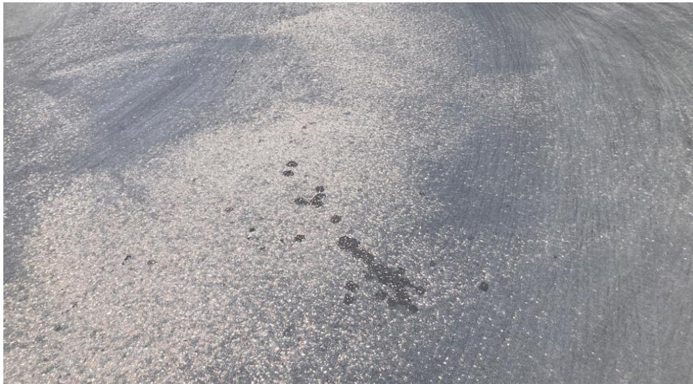
As asphalt ages and is trafficked extensively, the paving asphalt can wear and polish to a hazardous state. Crimped finishes and wearing layers are worn to a flat, smooth, shiny surface that is slippery when wet.
