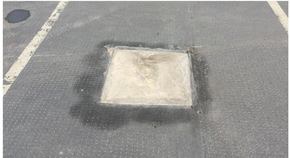
Patch repairs are commonly seen in asphalt substrates and although there are complex methodologies for such repairs, these seem rarely followed. Shrinkage related failures regularly occur with cracks opening at the perimeter of the repair, allowing water ingress.
