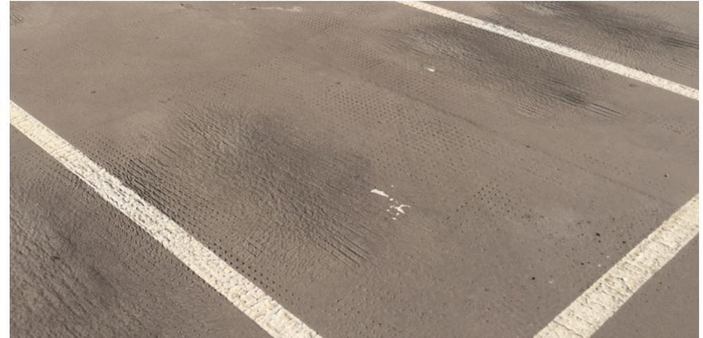
Mastic asphalt consists of limestone aggregates historically bound together by Trinidad Lake asphalt, but now by bitumen, or polymer modified bitumen.
