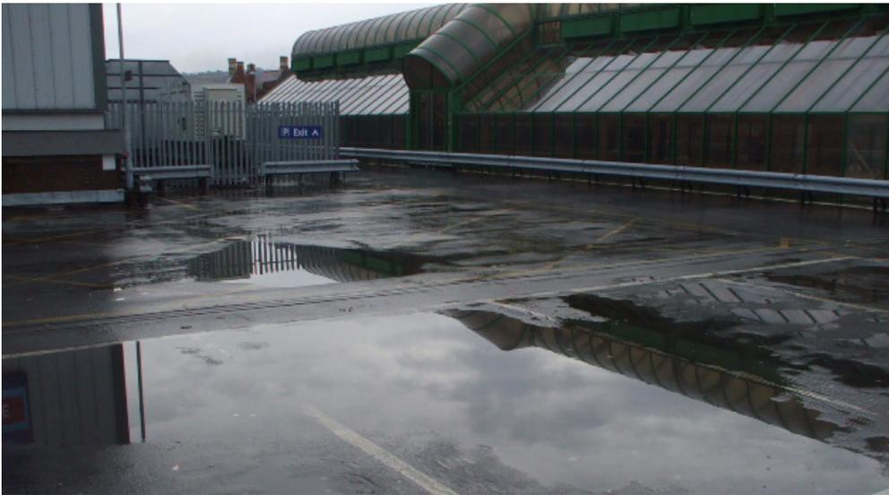
It is recommended that falls in car park decks should be a minimum of 1:60. Unfortunately, the designed and as-built construction do not always match, and ponding is common on asphalted car parks. Causes include poor construction, deflection within the structure, insufficiently designed falls and a lack of or poorly located drainage outlets.
