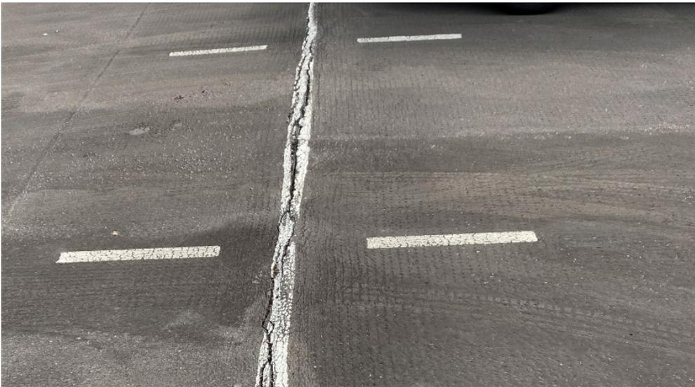
Cracks in the waterproofing allow a direct path for water and chloride ingress as well as carbonation. They most commonly occur in the weaker asphalt day joints or at upstands and interface details. Large car park structures will have numerous asphalt day joints and details creating a significant number of high risk zones.
