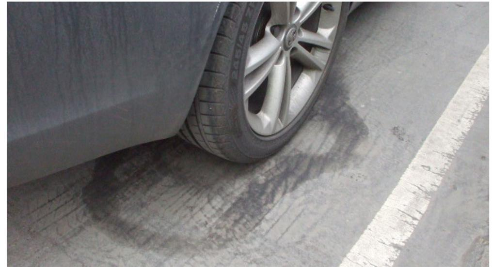
Where asphalt lacks enough stone content at the surface or is soft, tyre impressions or wheel indentations commonly form. As heavier electric vehicles increase in number, and temperatures rise due to climate change, the frequency of these will increase. Asphalt surfaces are softer where the ratio of bitumen-rich material to aggregate is higher. This can be due to variations in the size or amount of aggregate in the paving grade wearing layer or a paving asphalt layer which is applied too hot.
