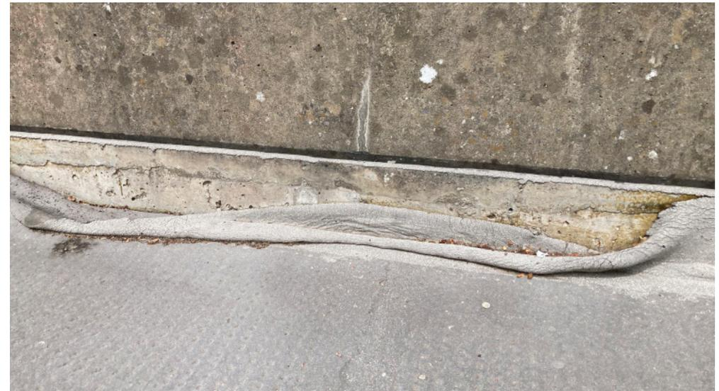
High thermal loads cause thermoplastic asphalt to soften, particularly the roofing grade mastic asphalt exposed at details. South facing aspects, or surfaces where heat or sunlight is reflected from buildings are especially vulnerable. Softened asphalt becomes mobile and will slump, especially on vertical details such as upstands and stair risers.
