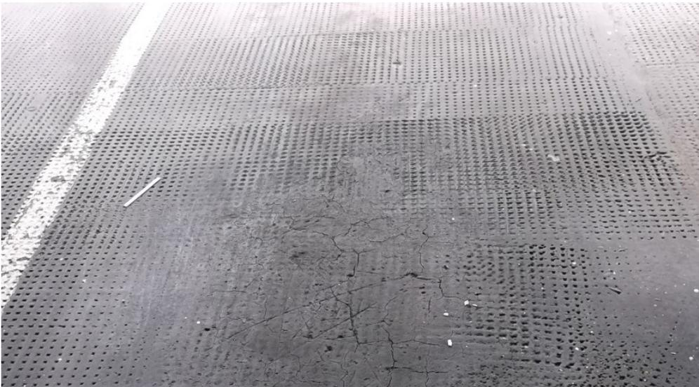
Fuel, oil deposits and other contaminants can attack the bitumen-based asphalt. This causes it to lose its physical and mechanical properties leading to degradation and even break up.
