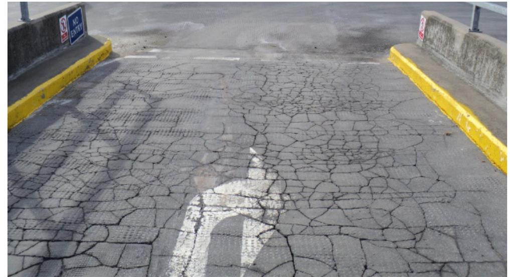
Alternatively, if the separating tissue between the asphalt and underlying concrete is damaged or missing, the asphalt may stick to the concrete. As the asphalt is designed to allow movement during temperature changes, it may tear and crack if adhered to the substrate. Similarly, cracking and movement in the underlying concrete transfers directly into the asphalt, resulting in crack formation in the asphalt.
