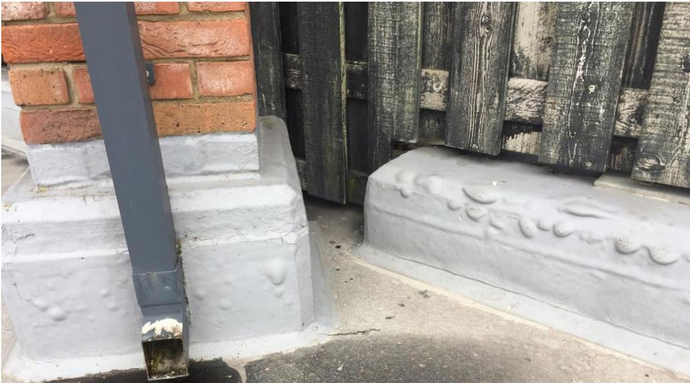
Roofing grade mastic asphalt is used to form interfaces with other details. All of these details whether upstands, drainage outlets, channels, posts, or plinths etc. are potential failure points for asphalt waterproofing.
