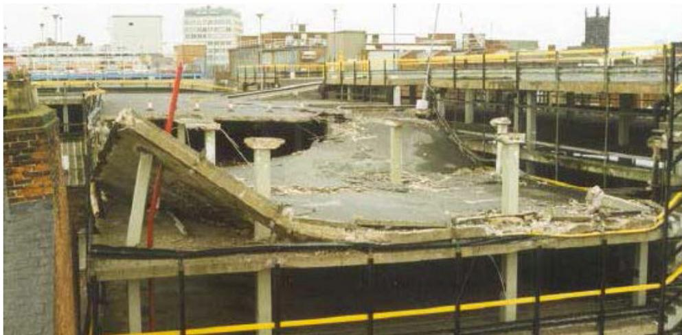
Pipers Row car park, Wolverhampton in 1997. Partial collapse attributed to carbonation and a lack of waterproofing to cracks <https://www.hse.gov.uk/research/misc/index.htm>
